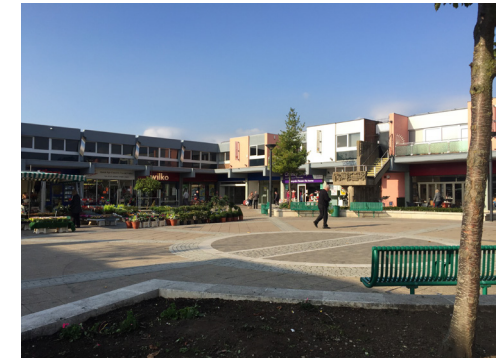
Fig 1.1: The existing central market square
